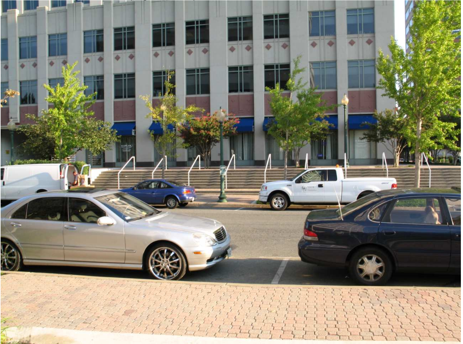
Left Side of Building: South Face (August 31, 2010)
