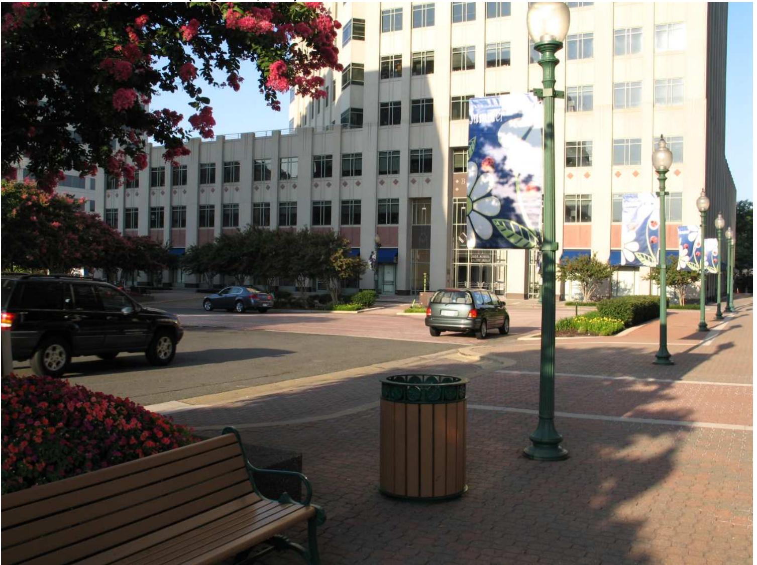
Front of Building : East Face (August 31, 2010)
